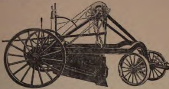
The Maney Four-wheel Scraper. Figure 8.
